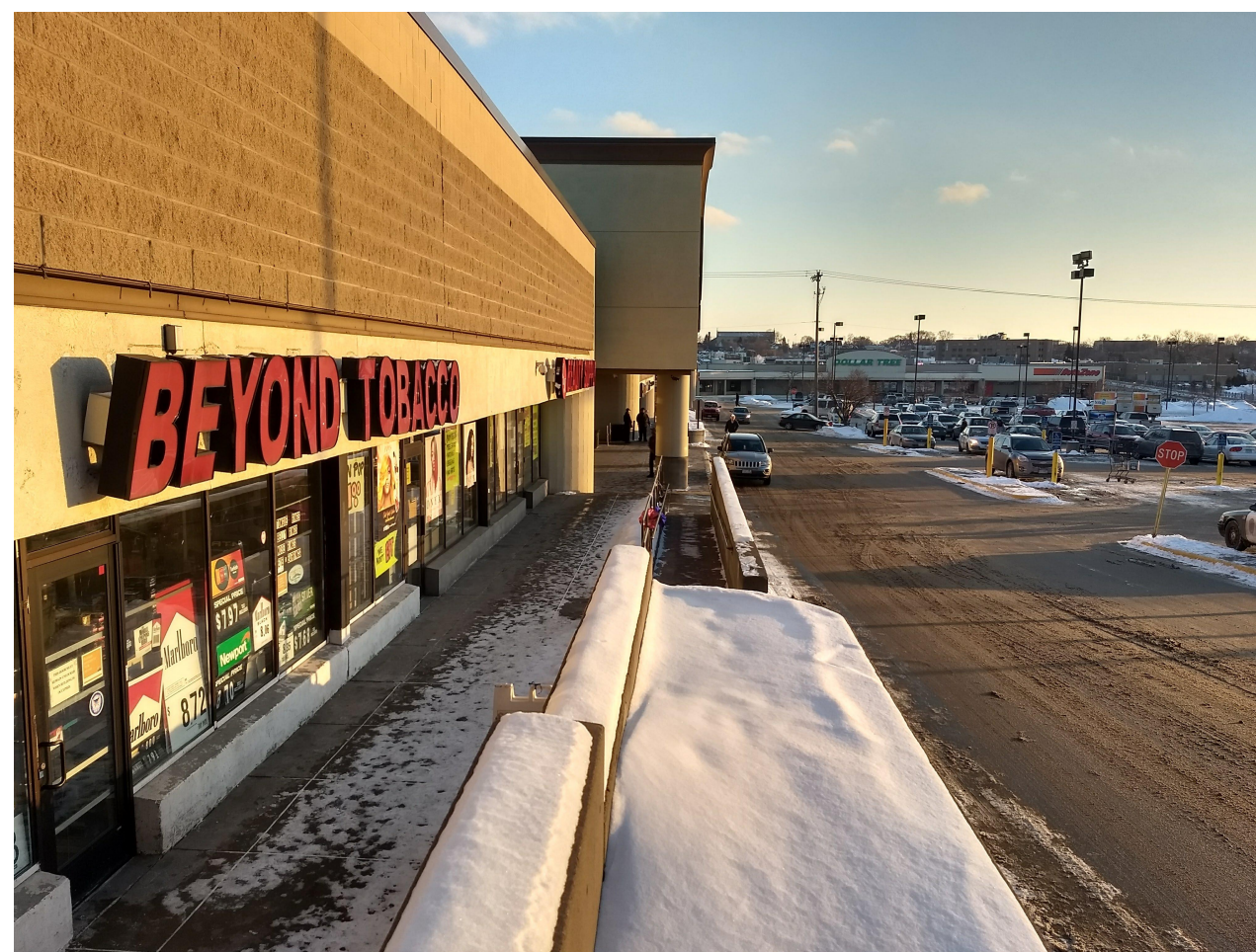
LOOKING SOUTH FROM NORTH END OF SITE
