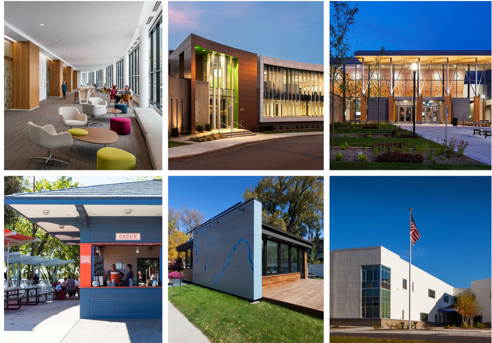
Top left to bottom right: Be The Match; DC Group Office Headquarters; Fireman's Park & Chaska Curling and Event Center; Sandcastle; South Minneapolis Office; and Twin Cities Academy
