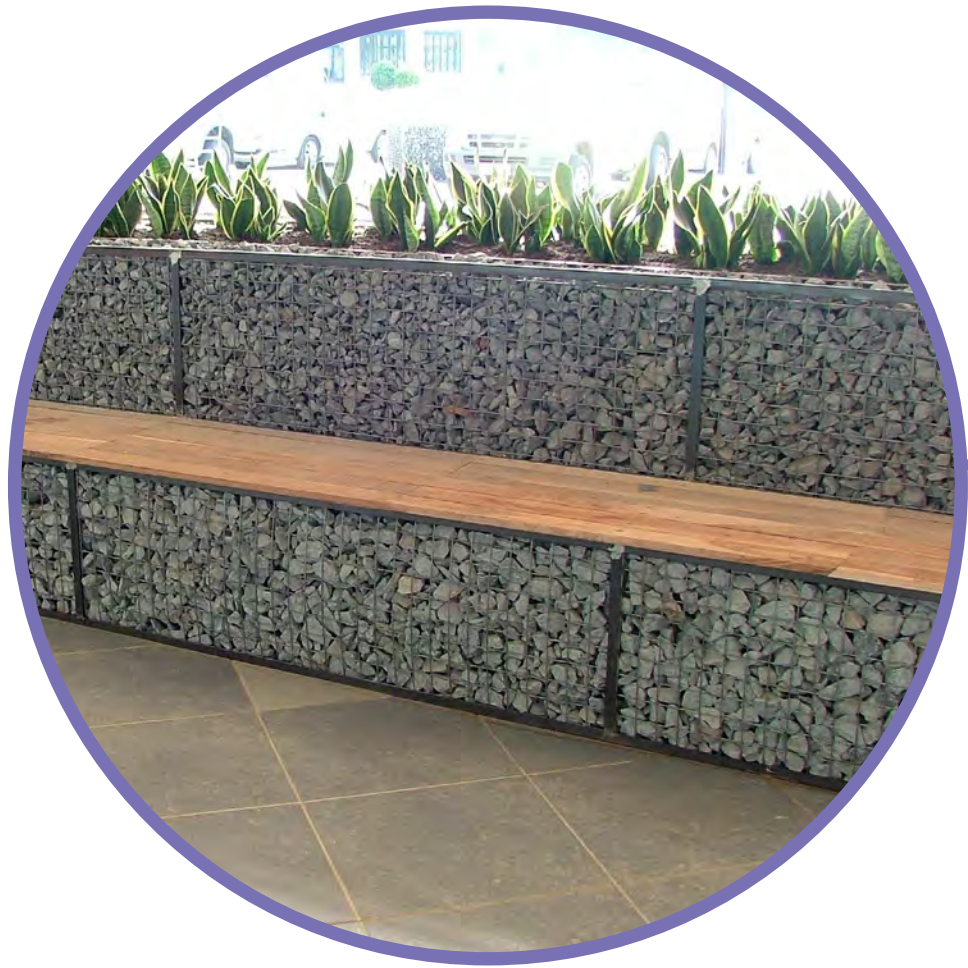
GABION WALL - RECYCLED MATERIAL FILL - MULTI-FUNCTION SEATING - SPACE-DEFINING GREEN SPACE
